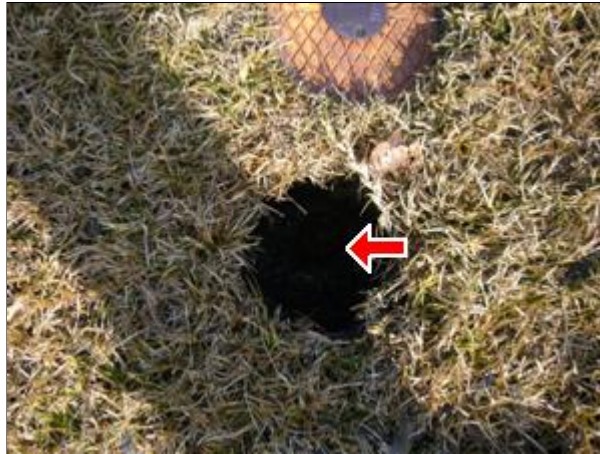
8.3 Picture 1 Main water shut off valve
