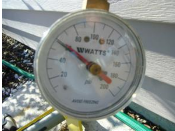
8.4 Picture 1 Water pressure test
