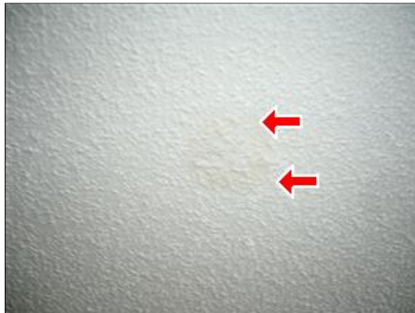
5.0.D Picture 1 Repaired spot
