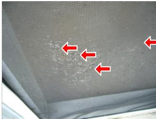
2.3 Picture 2 Holes in screen
