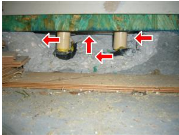
3.2 Picture 1 Exposed water pipes
