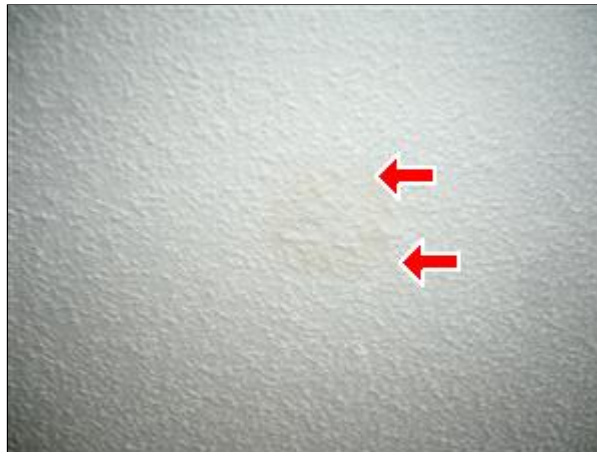
5.0.D Picture 1 Repaired spot
